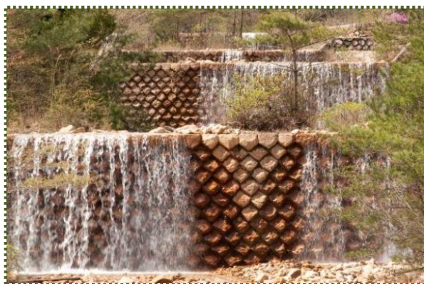
写真-3 鍍積堰堤
