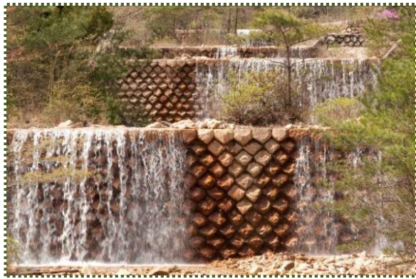
写真-3 鍍積堰堤
